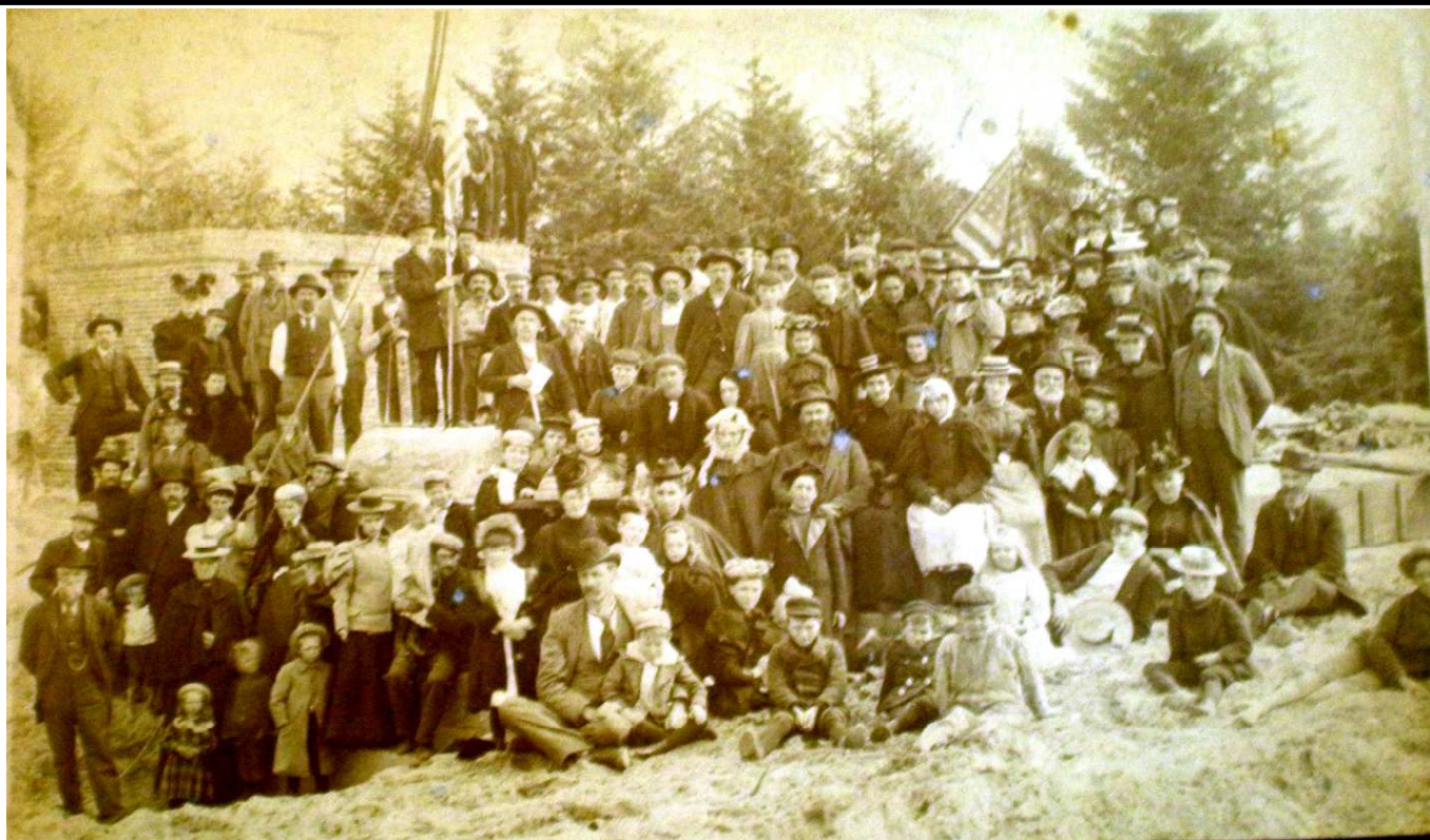
Gray's Harbor Light House, Laying the corner stone, Aug. 23 rd 1897.
